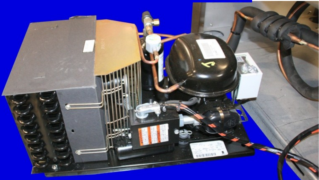
Illustration 2.B RUT050-PM Condensing Unit Assembly
