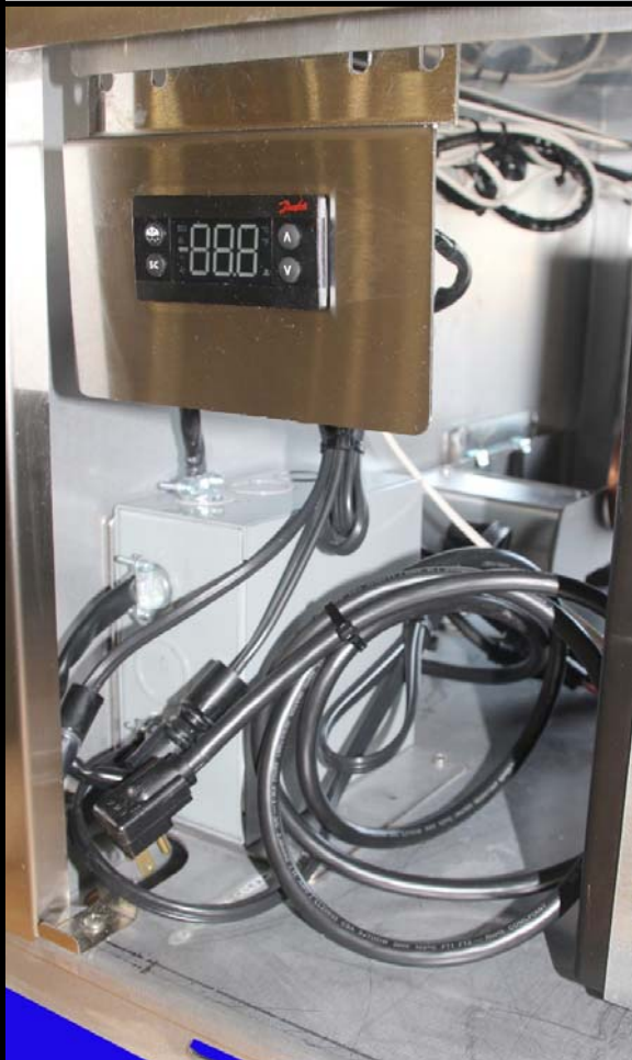
Illustration 2.A: RWTT65-PM(L) Electronic Controller Assembly
