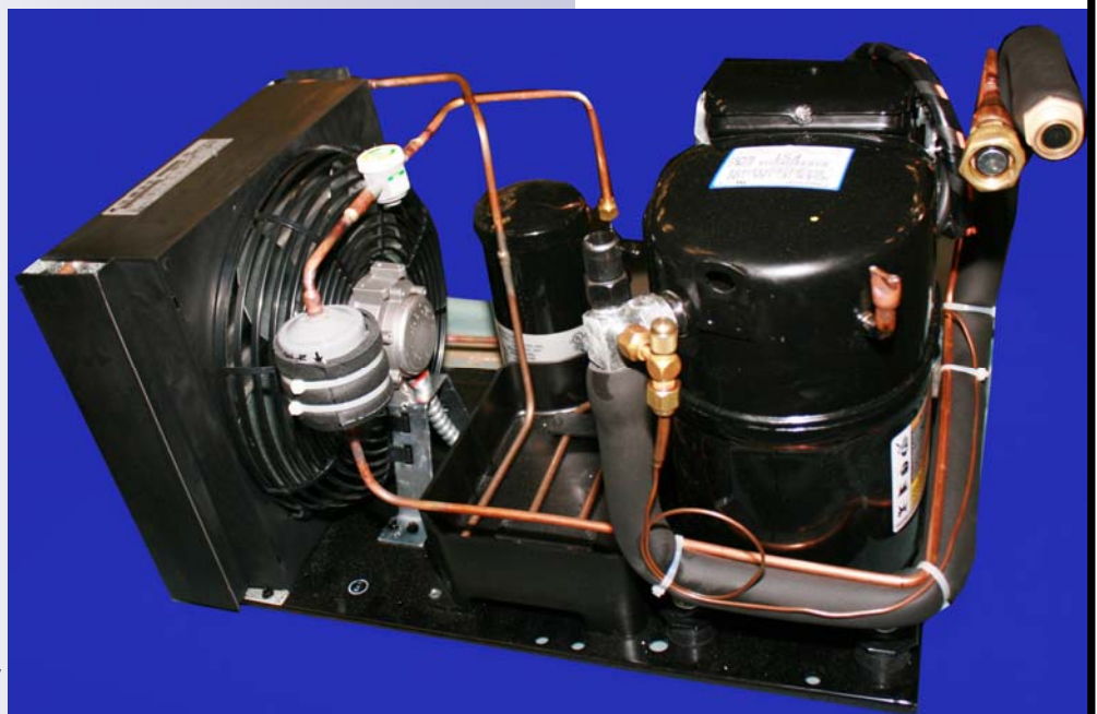
Illustration 2.B: RUT520-2-PM Condensing Unit Assembly
