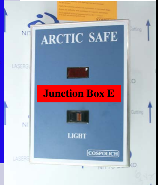
Illustration 2.C: LED Digital Temperature Read-out and Light Switch, Junction Box E
