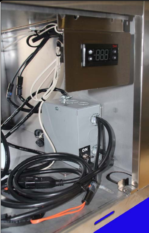
Illustration 2.A: RWTT65-PM(L) Electronic Controller Assembly
