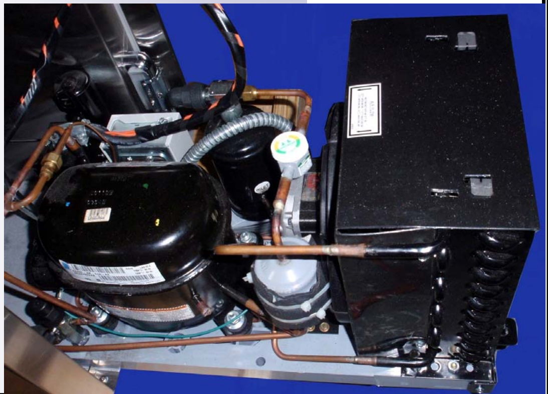
Illustration 2.B- Condensing Unit Assembly
