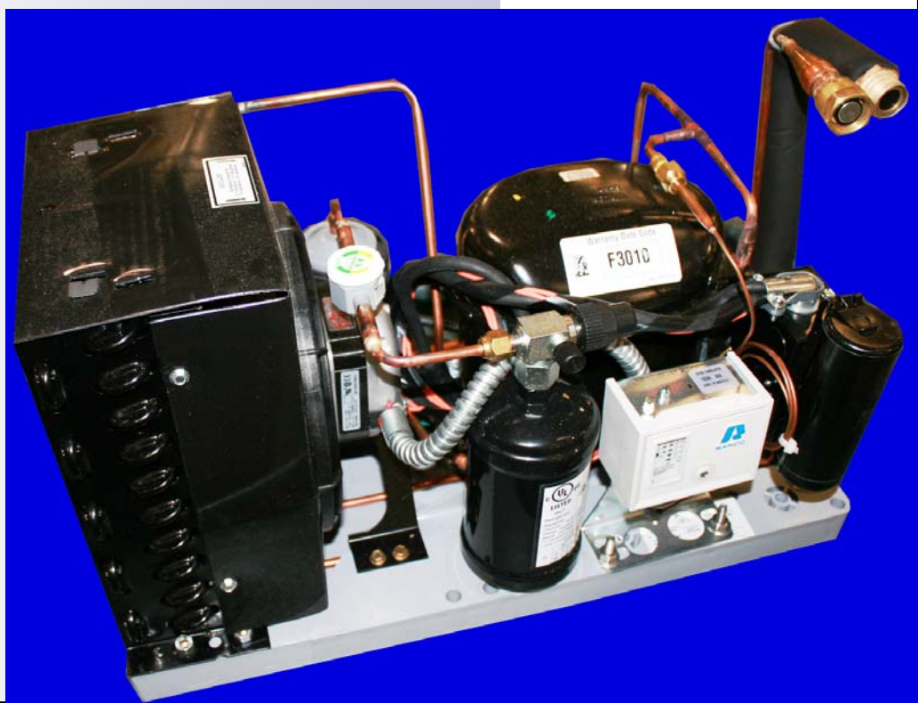
Illustration 2.B: RUT220-PM Condensing Unit Assembly
