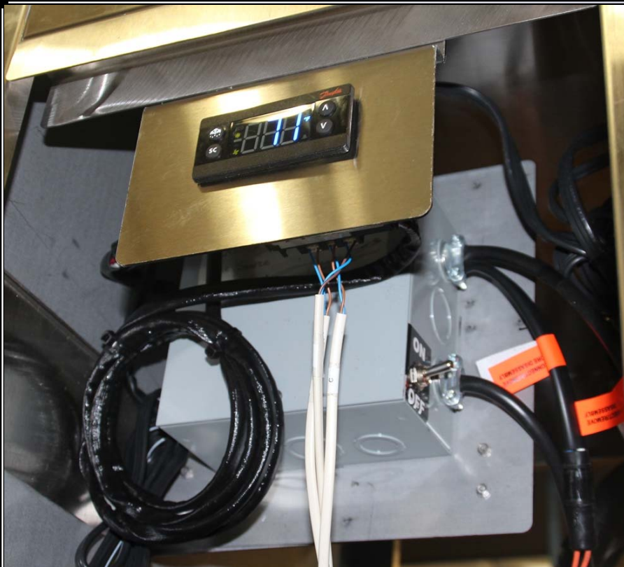
Illustration 2.A: RWTT65-PM Electronic Controller Assembly
