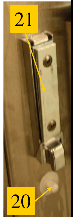
Illustration 7.I-Door Latch Strike Detail
