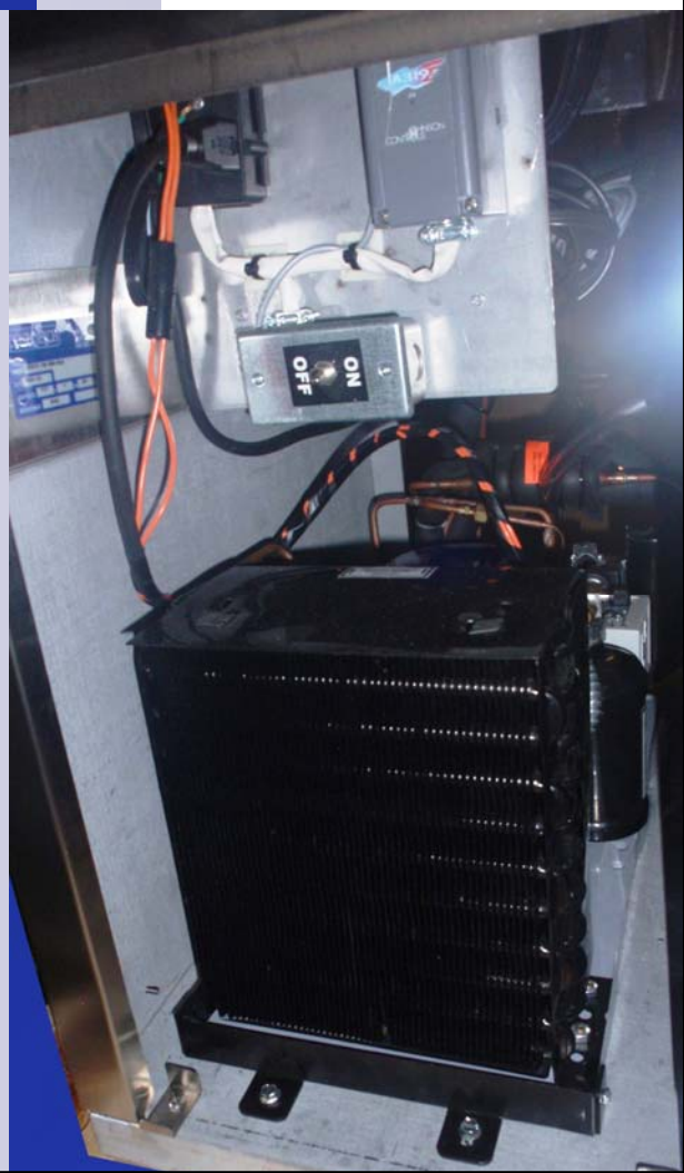
Illustration 2B-Control Panel & Condensing Unit Assemblies
