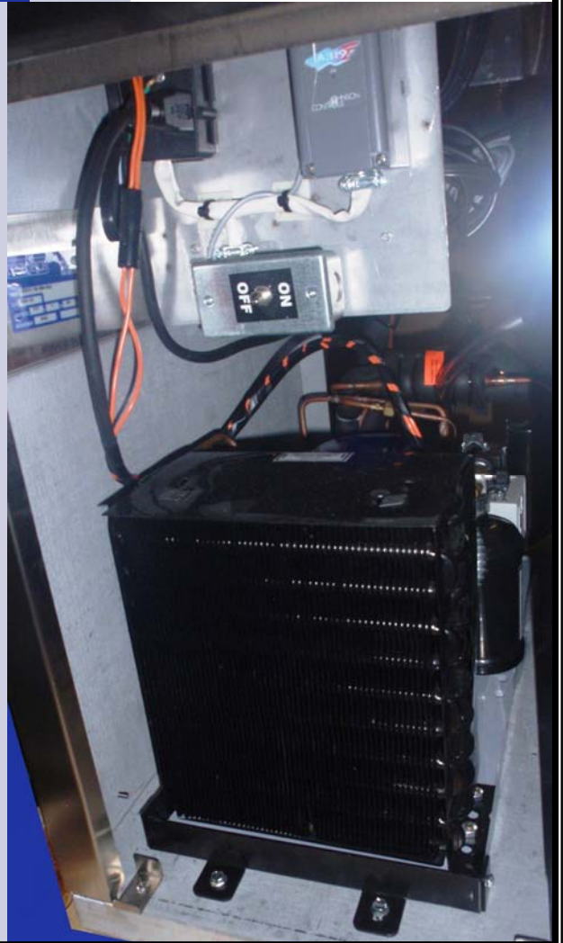
Illustration 2.B-Control Panel & Condensing Unit Assemblies
