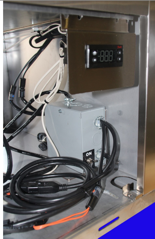
Illustration 2.1B: R10 Series RWTL651-PM(L) Prepped Electronic Controller Assembly
