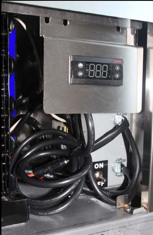
Illustration 2.A- Electronic Controller Assembly
