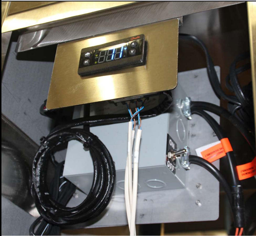
Illustration 2.A: RWTT65-PM, Electronic Controller Assembly
