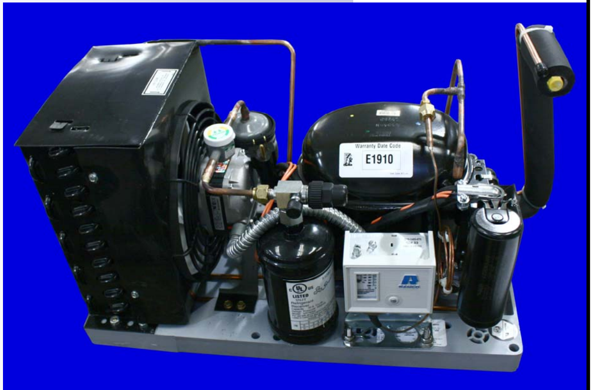
Illustration 2.B: RUT220-P, Condensing Unit Assembly
