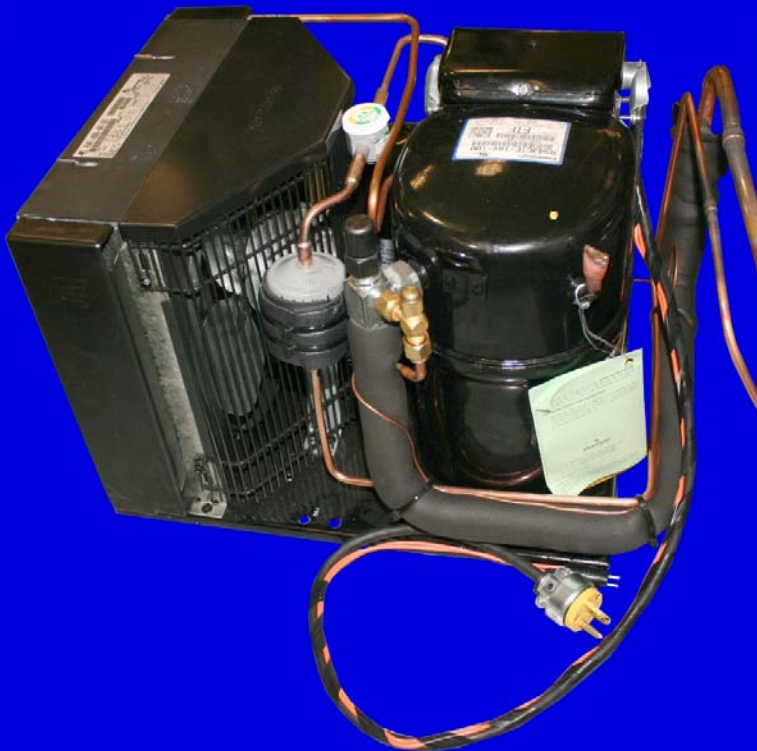
Illustration 2B RUT550-P Condensing Unit Assembly
