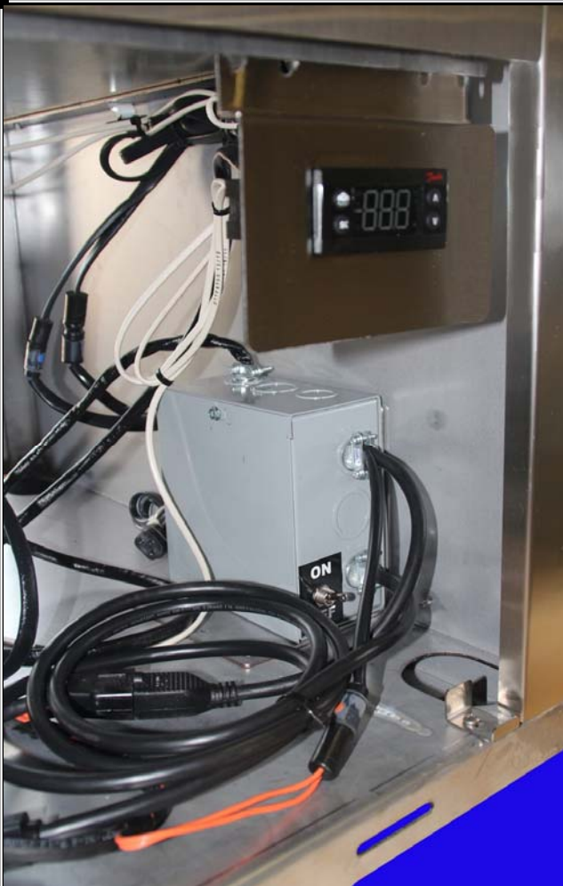
Illustration 2.A: RWTT65-PM(L) Electronic Controller Assembly
